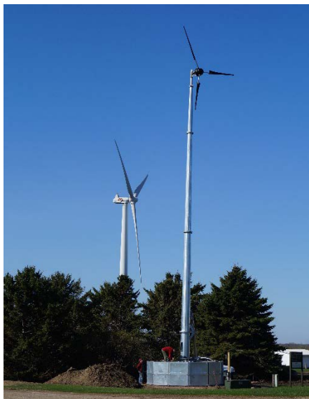
Figure 4. South 10 kW Wind Turbine Installed
