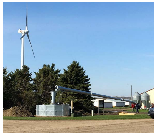
Figure 3. South Tower Folded Down for Turbine Installation
