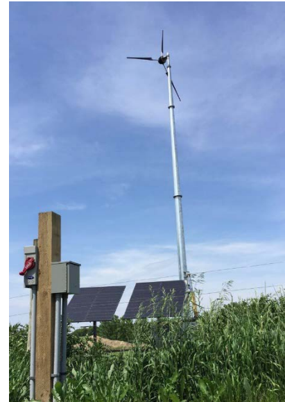
Figure 2. North Wind Turbine with 4kW Pole-Mounted Solar Array
