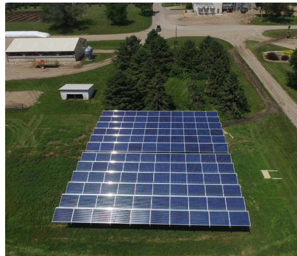
Figure 1. tenKsolar 50 kW Solar PV Array
